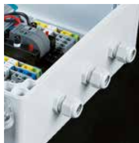
Incoming/Outgoing cables M20 cable glands
